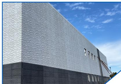
**Block 9 Tower & Parking Structure** - Fargo, ND: Wells manufactured and erected nearly 220,000 combined sq. ft. of precast product between the two projects out of our Grand Forks, Albany, and Rosemount production facilities. The 1,690 precast concrete members in the podium and tower include architectural solid precast components that showcase a beautiful sandblast finish with reveals.
