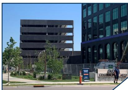
Wells also produced and erected precast for the 1,214-stall parking structure, which is a three-bay wide design with vertical vehicular circulation occurring in the center bay. The facades on all four sides are flat, and clad with integral color acid etch architectural precast.
